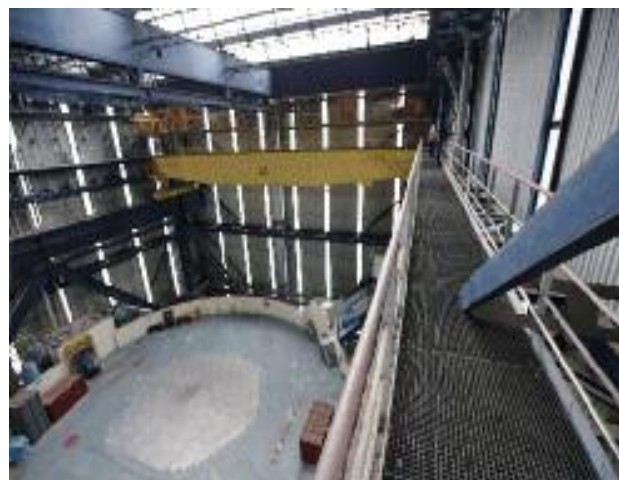
Bugey 1 dismantling worksite – UNGG gas-cooled reactor fuel loading zone – August 2011
